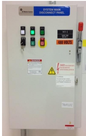
Power Distribution Box (aka A1 Main Disconnect)
